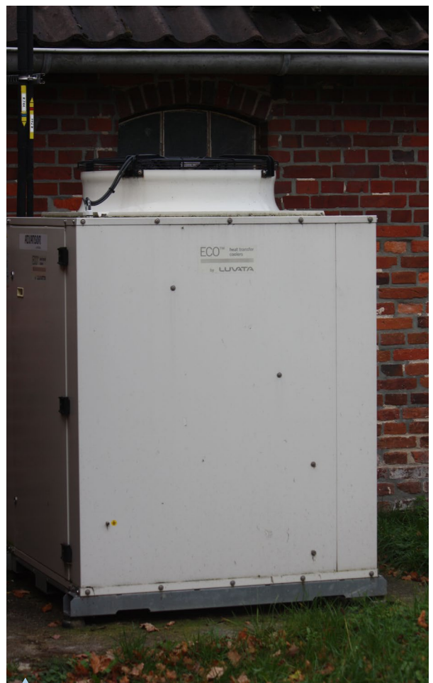
Cooling system for cooling cabinets, run with CO 2
