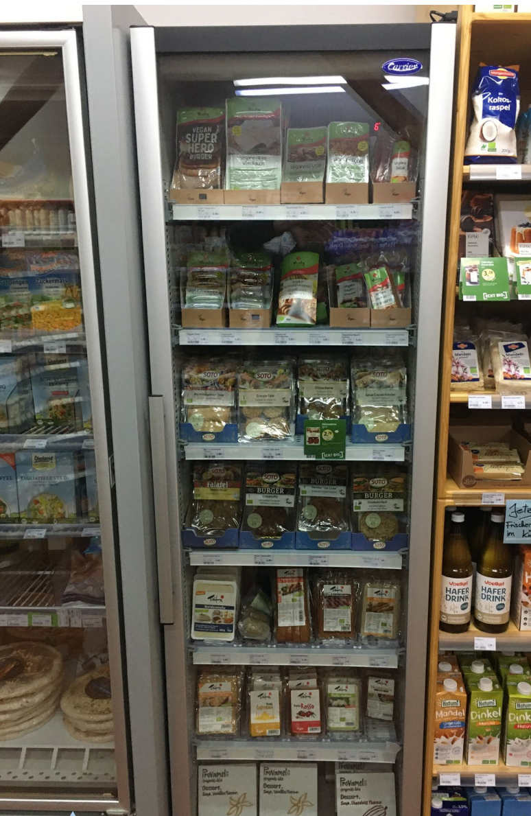
R600a-run cooling unit for vegetarian products.
