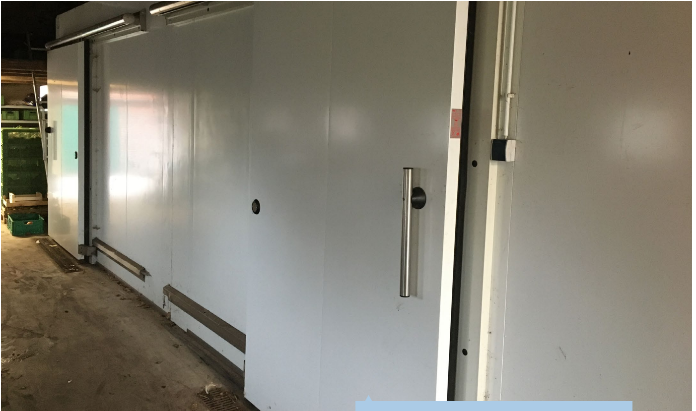
Cooling cabinets for fresh vegetables with three separate rooms capable of temperatures ranging from 2-12 °C (depending on the product).
