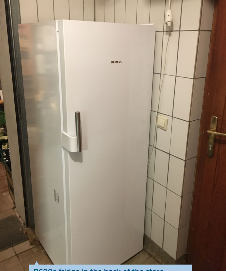
R600a fridge in the back of the store.
